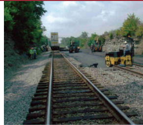
Above: Reconstruction of the foundation for a railroad track
