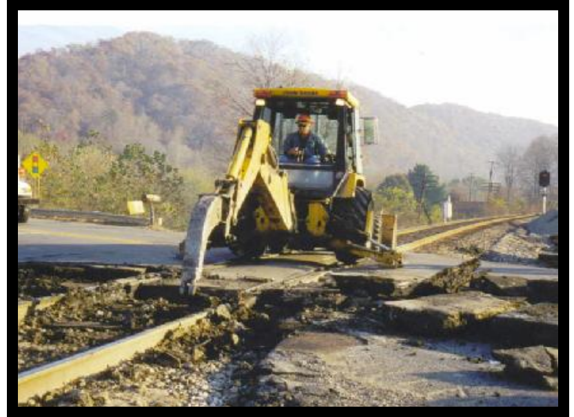
Removing old crossing 08:30
