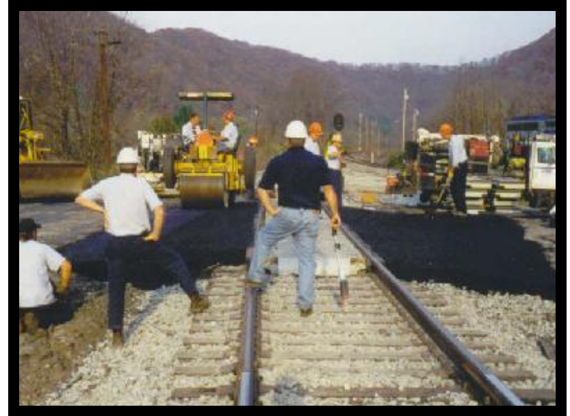
Compacting hand-spread approaches
