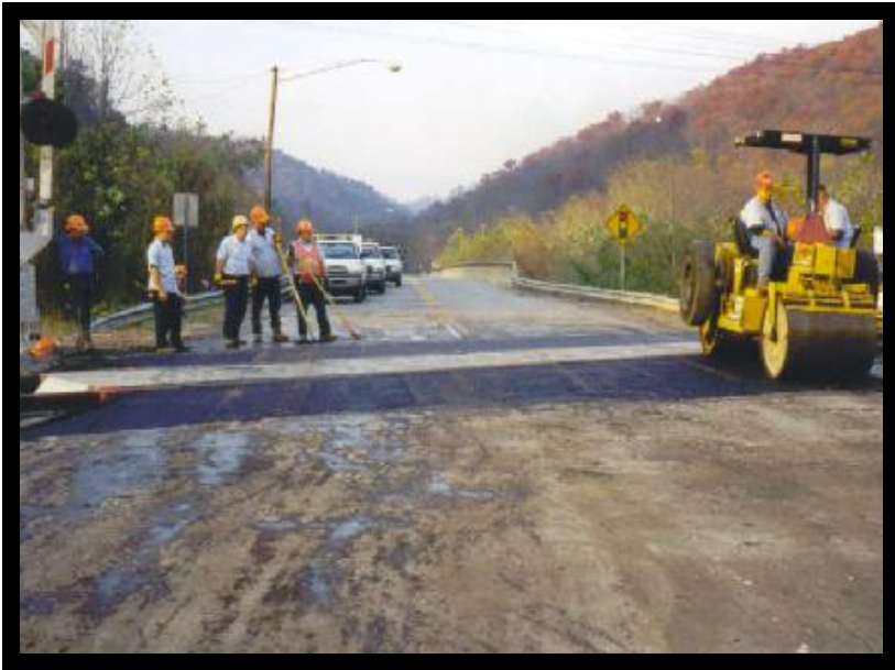
Finished compacting asphalt approaches 16:50
