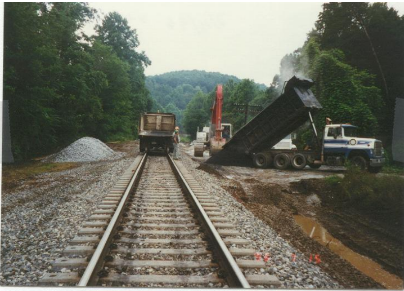
Unloading hot mix asphalt for transloading to hi-rail dump
