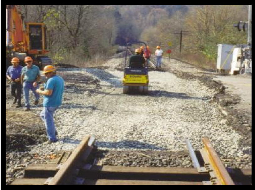
Compacting ballast 11:20
