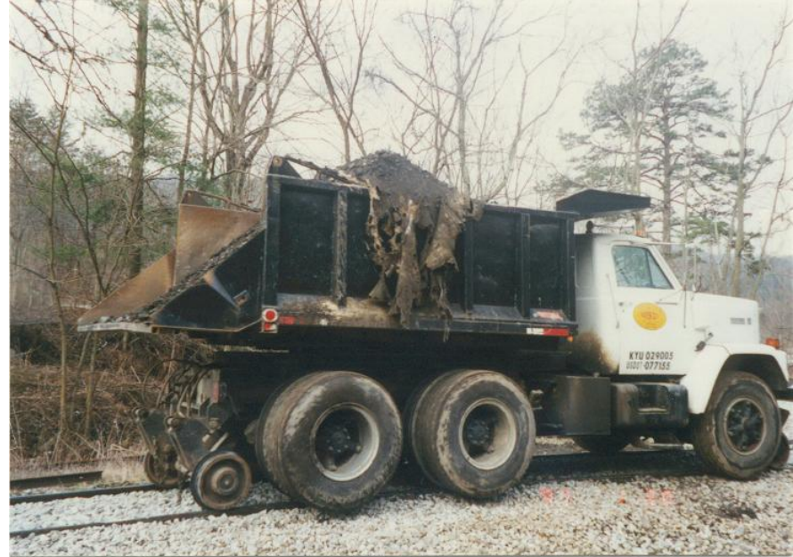
Hauling fouled ballast from tunnel
