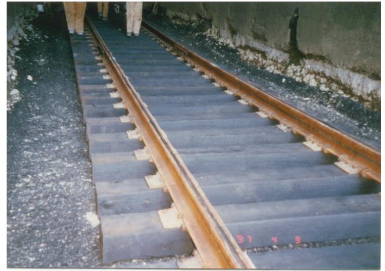
Wood panel on asphalt layer prior to adding ballast
