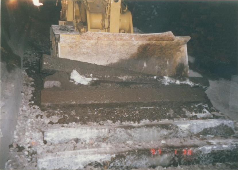
Removing track and location 2 (1/30/97)
