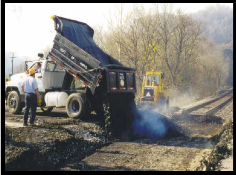
Dumping asphalt 10:15
