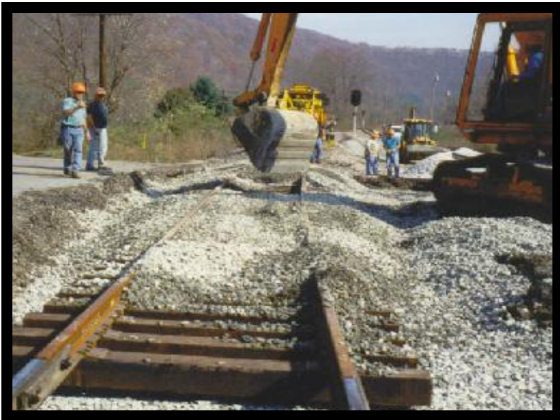
Spreading cribbing rock 11:30
