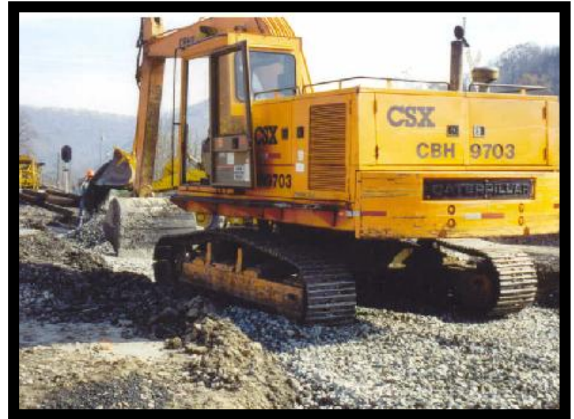
Dumping and spreading ballast
