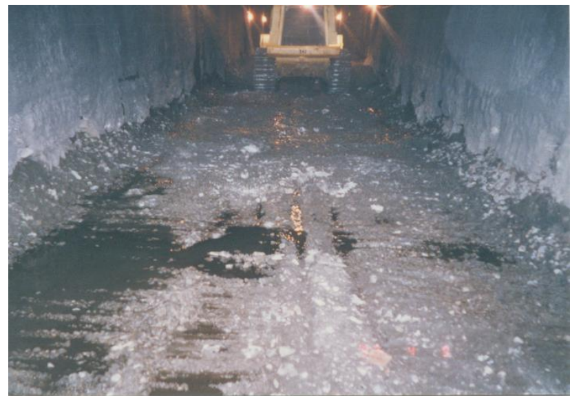
Excavating trackbed material
