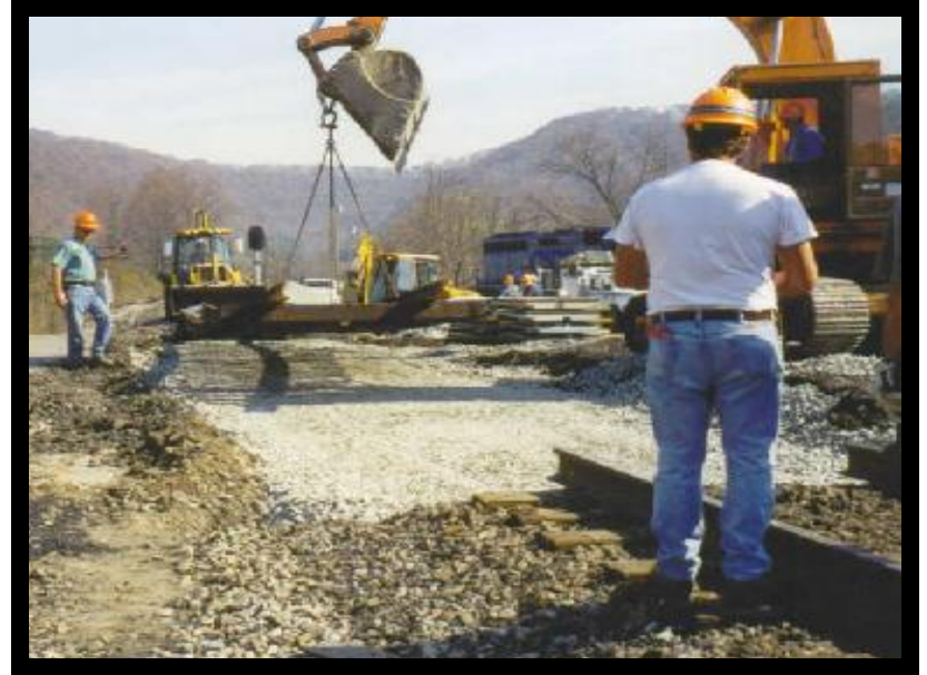
Positioning new panel
