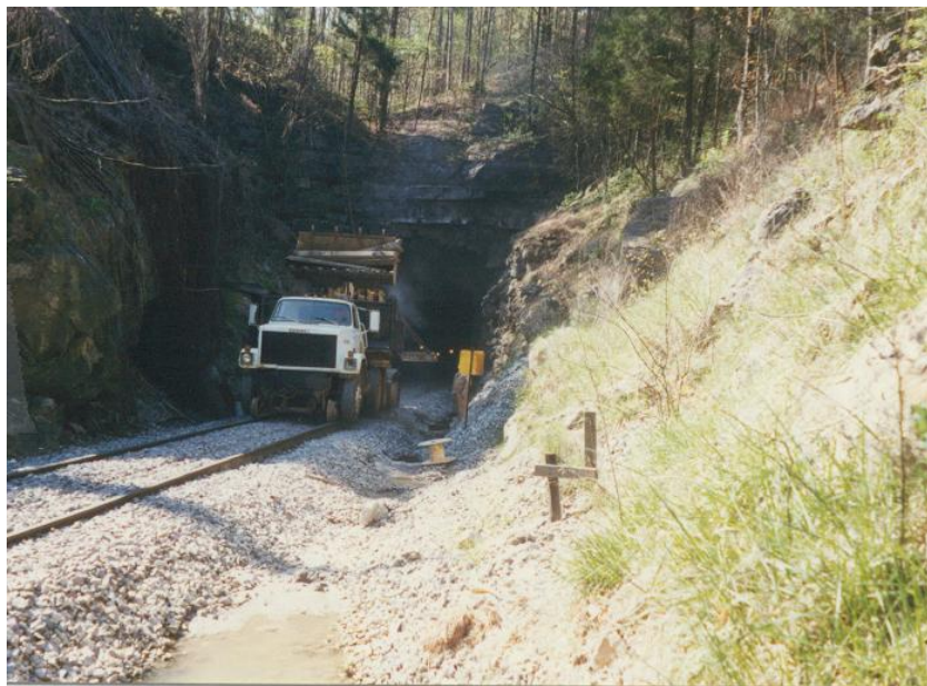
Loading steel ties and roadbed at north end
