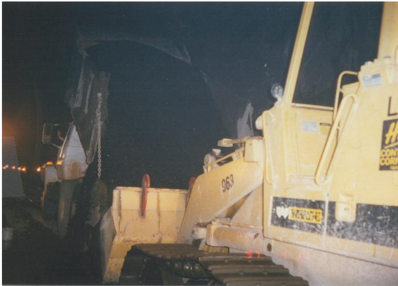
Unloading hot mix asphalt inside tunnel
