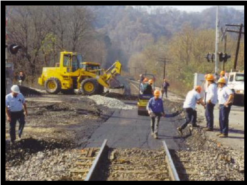
Compacting asphalt and dumping ballast
